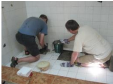
Don and Robert replacing tile in boys' washroom.
