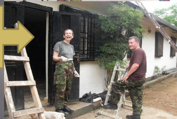
Painting parlour & repairing termite damage and roof drainage
